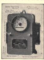
Fig. 16.—Polyphase watthour demand meter (Westinghouse Type RO).
